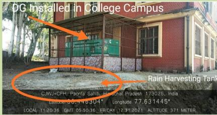
Yes, 1 Number of Genset - model, Sudhir, 100 kVA; Diesel type. Acoustic enclosure canopy and adequate stack height is under planning
